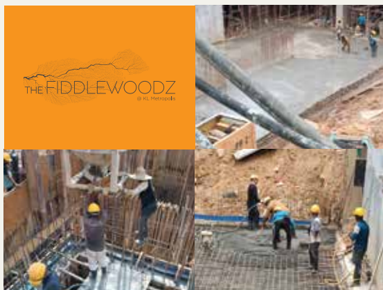
THE FIDDLEWOODZ @ KL METROPOLIS Progress Date | As of Q4 2022 Site Progress | 12% Expected Year of Completion | 2025
