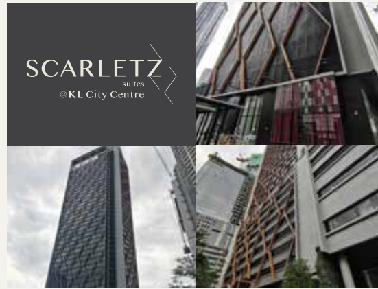
SCARLETZ SUITES @ KL CITY CENTRE Progress Date | As of Q3 2022 Site Progress | 100% Year of Completion | July 2022
