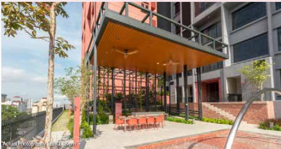
Actual Photography | Grand Entrance
