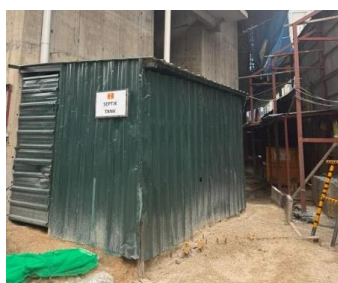
Repurpose old zinc metal deck as a septic tank storage.
